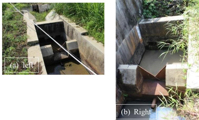
**Figure 6.** V-notch weir cannot measure the seepage discharge (both on the left and right of the dam).
