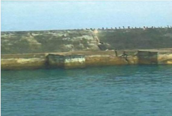
**Figure 2.** Cracking on breakwater concrete wall after an earthquake on January 21<sup>st</sup>, 2012.
