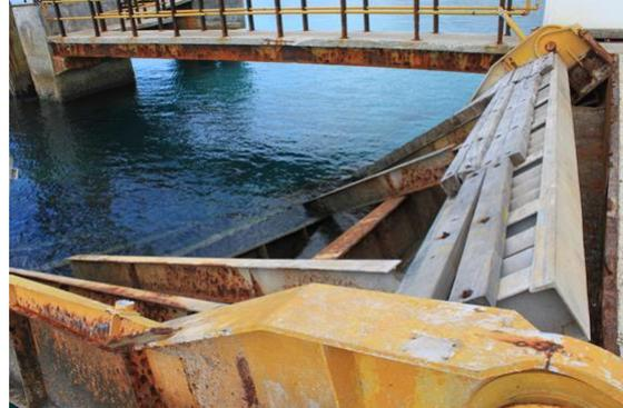
**Figure 5.** Major damage on movable bridge after Lua storm on March 2012.
