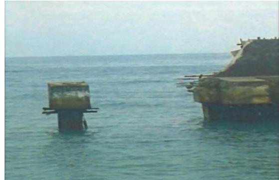
**Figure 3.** Significant damage of breakwater due to high wave on January 25<sup>th</sup>, 2012
